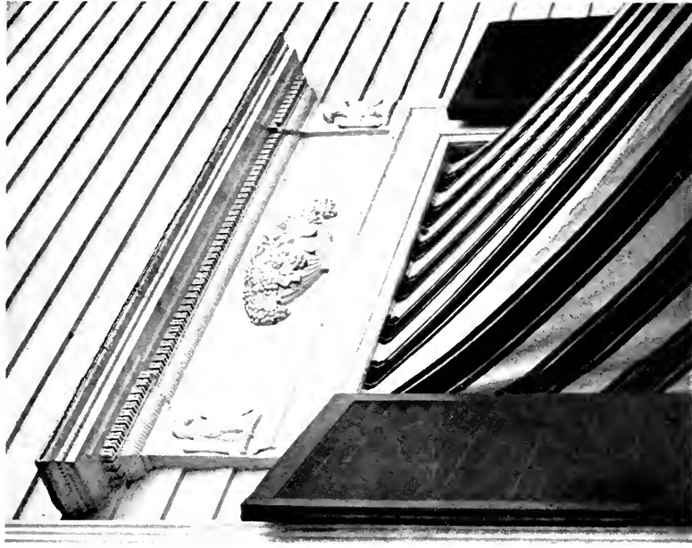
PLATE XVII.—Keyed Marble Lintel, Peabody-Silbee House; Entablature of Window Frame, "Oak Hill."
